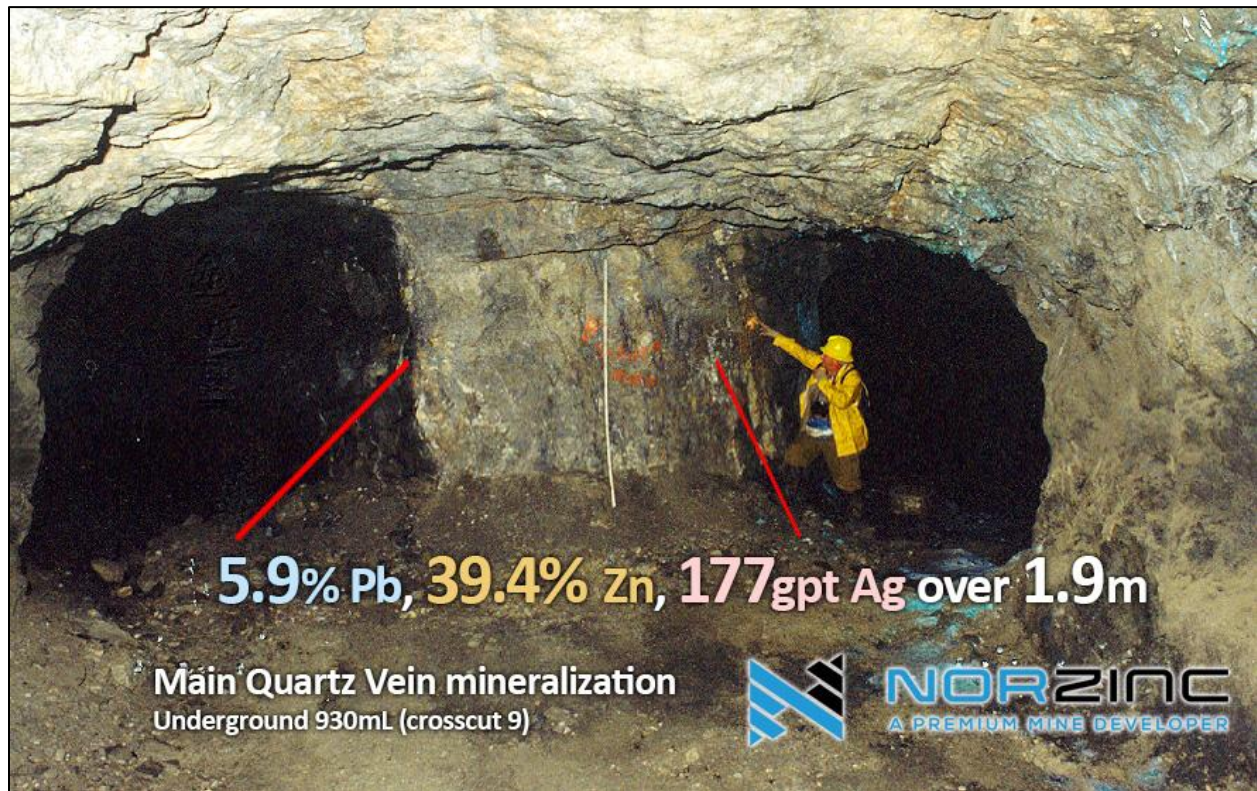
Figure 7-4: MQV Exposed Underground
